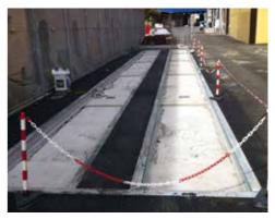
Example of an installation on an asphalt weighing surface
